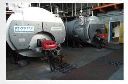
**MCB Civils** were the main contractor for the demolition and site clearance of the former Tyrone County Hospital site in Omagh. The practitioner was keen to see if the RMS could find solutions for the wide range of resources that would become available during the demolition works and clearance of such a large site. Among the resources identified were 2off oil fired 3000 kg/h 10 bar steam boilers. These had been planned to be disposed of as scrap metal waste.
