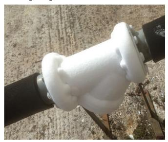
The refrigeration system has to deal not only with thermal gains to the space being cooled, there are heat gains to the pipework that must be considered. The suction low pressure liquid lines must be insulated to prevent excessive heat gain prior to evaporation and the suction lines must be insulated to prevent excessive un-useful superheat.
